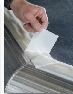
8 Peel off the protective release liner.
