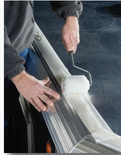
7 Roll down with a soft roller to conform over contours, seam edges, rivets, or screw heads.
